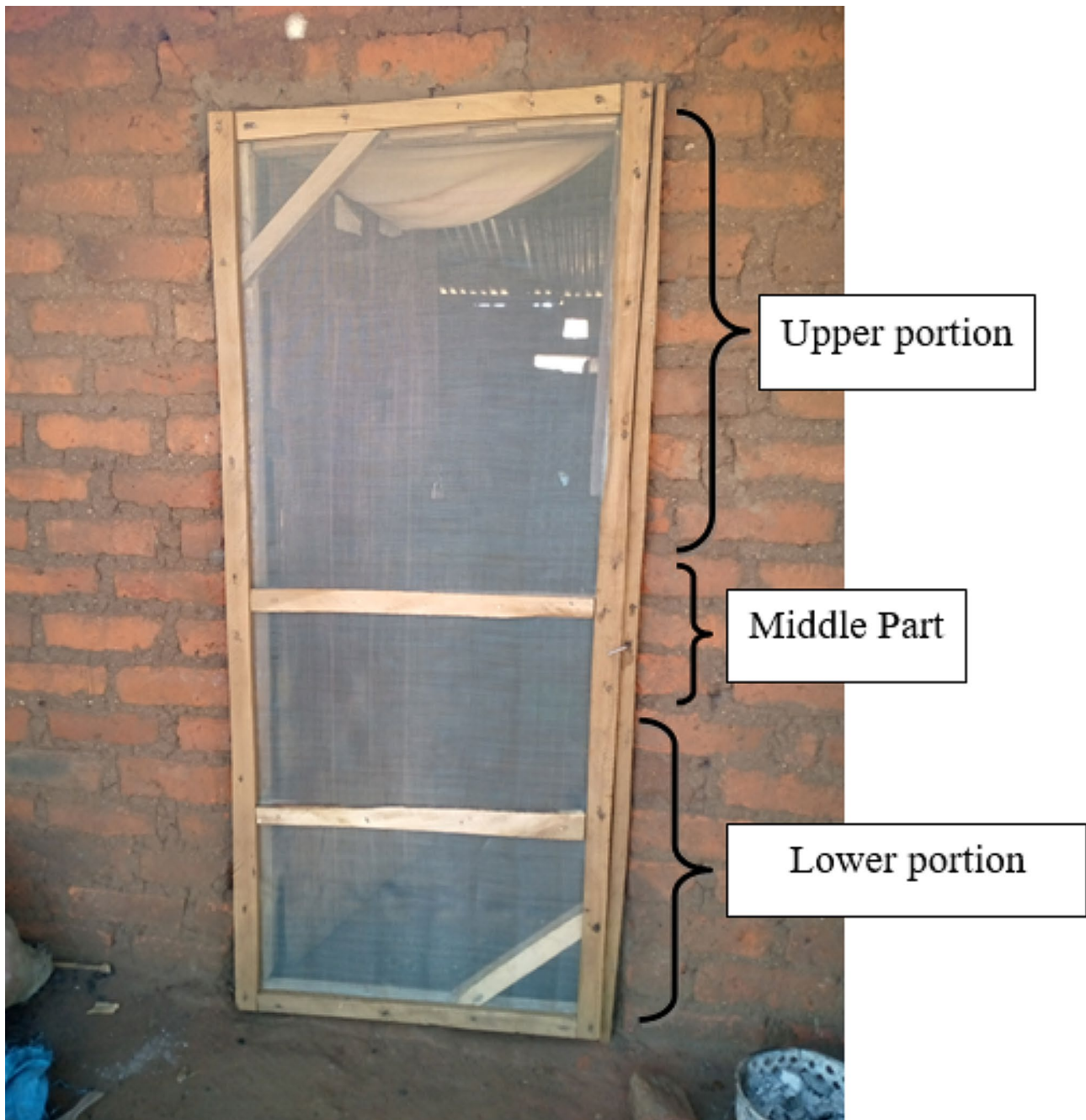
Fig. 2 A newly installed door screen showing the three portions considered in the questionnaire to assess damage
