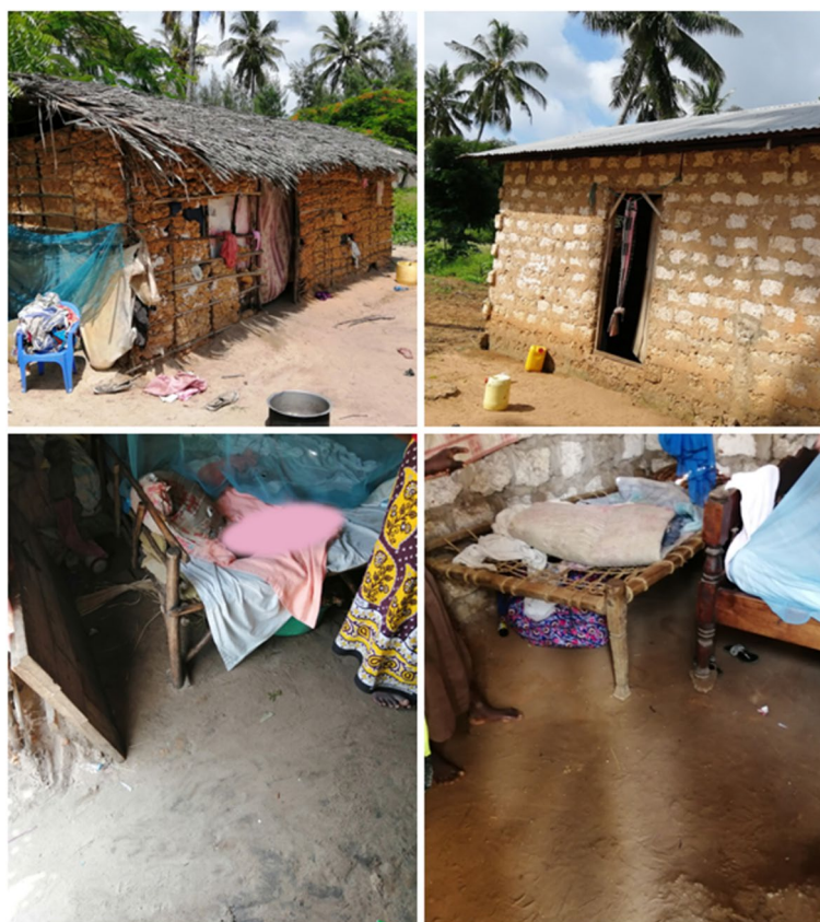
Fig. 1 Typical rural mud and brick houses with their unsealed earthen floors in the study area in coastal Kenya
