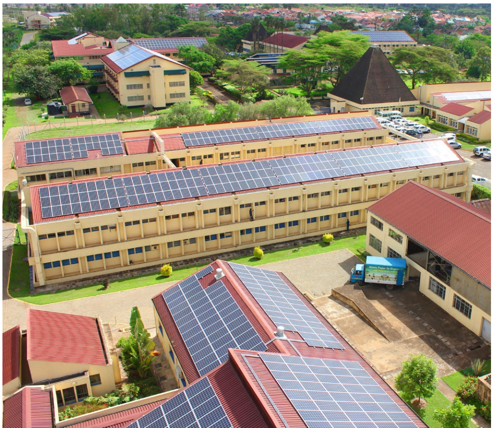
A semi-aerial view of the icipe Duduville Campus headquarters. A total of 3658 PV modules have been installed on rooftops on both icipe campuses. Photovoltaic modules placed on roofs have various advantages, for instance, better use of available space and natural cooling of the spaces underneath.
