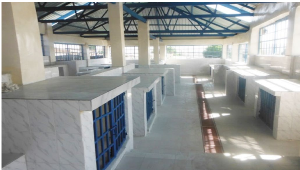
View from inside Gobanimo Market after rehabilitation
