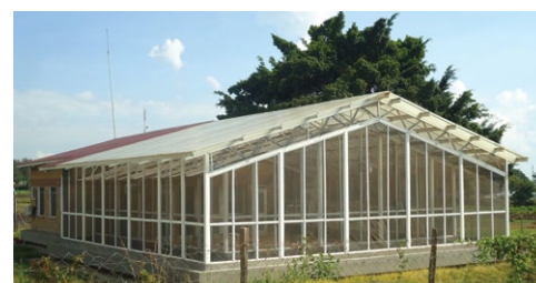
Bottom: New mosquito containment facility.
