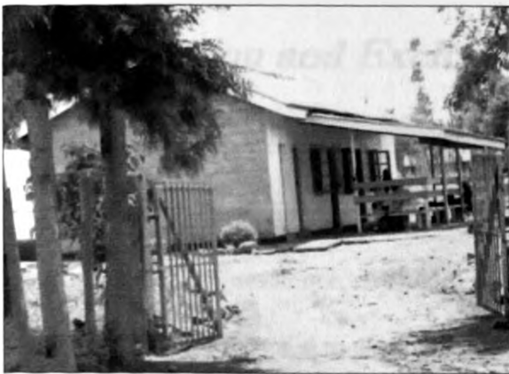
PLATE 3.2 – THIBA HEALTH CENTRE NEAR WANG'URU (MWEA). THIS IS A GOVERNMENT INSTITUTION
