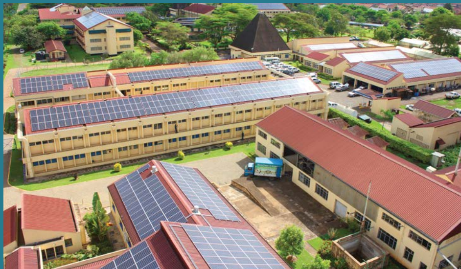
A semi-aerial view of the icipe Headquarters at Duduville. A total of 4130 PV modules have been installed on rooftops on both icipe campuses. Photovoltaic modules placed on roofs have various advantages; for instance, better use of available space and natural cooling of the spaces underneath.
