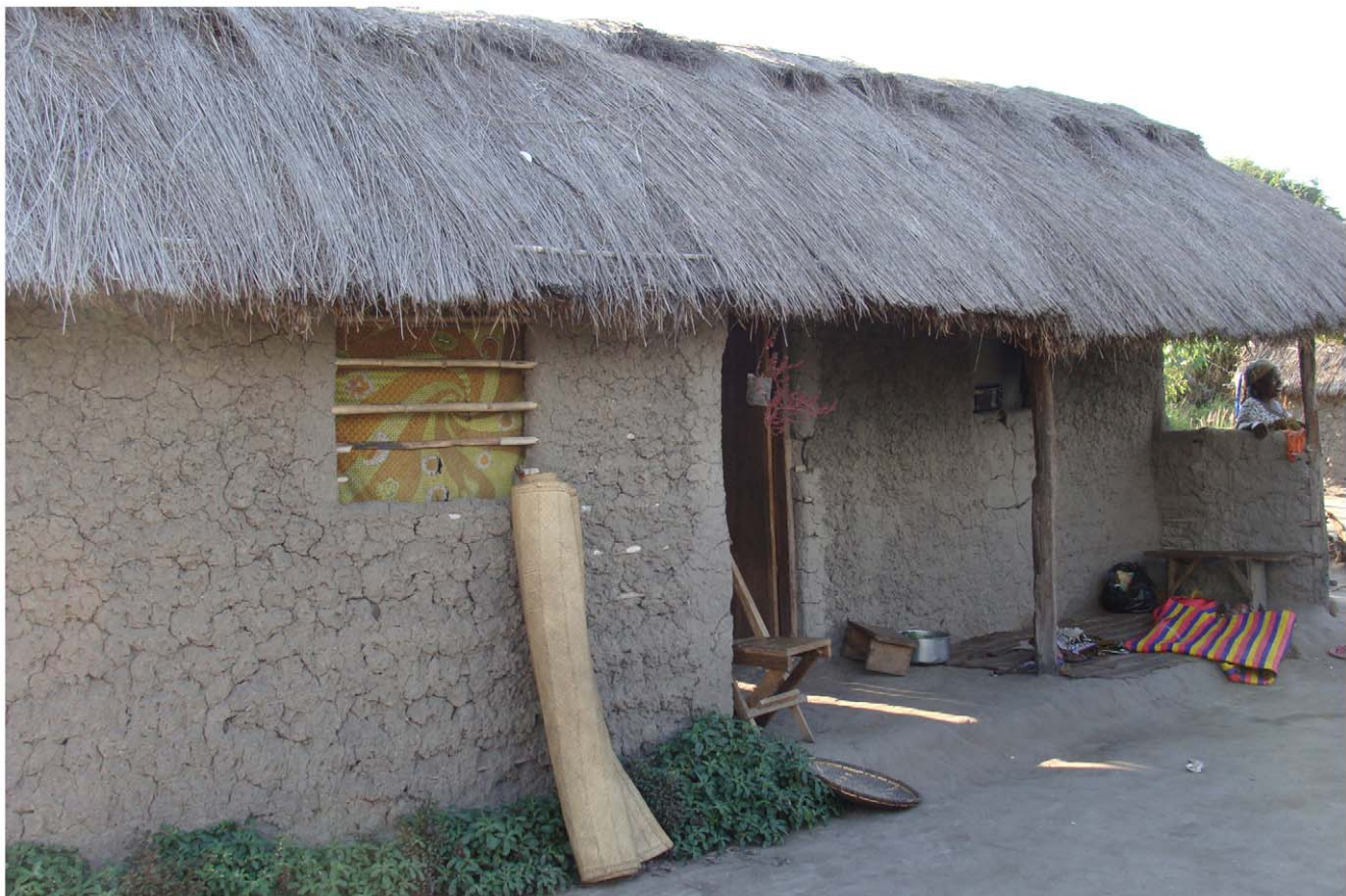
Figure 1. A local house. The local houses are made of mud walls and thatched roofs. They have one door and two windows and open eaves (open spaces between the roof and the wall). doi:10.1371/journal.pntd.0000773.g001
