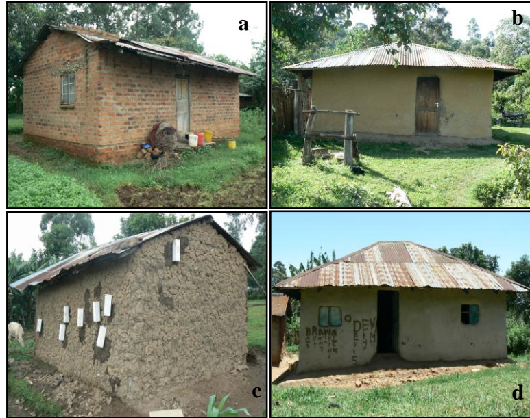
Plate 5.5: Four different wall substrata recorded in human house at homestead. a) Bricked cemented wall; b) Muddy wall smoothed with mud; c) Muddy wall not smoothed and d) Muddy wall smoothed with mixture of mud and cow dung
