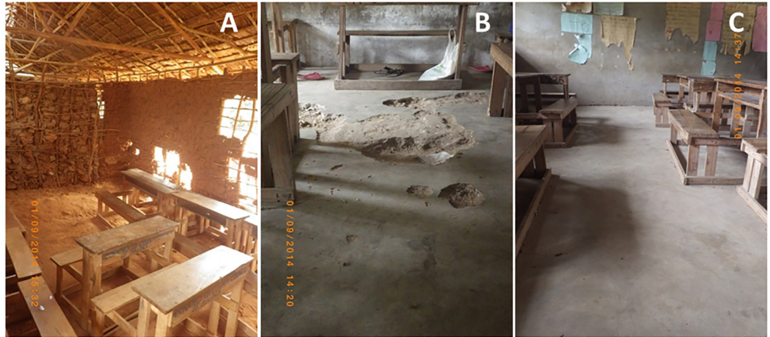
Fig 1. Examples of school classroom floors. (A) Natural sand/soil (MS2). (B) Cracked concrete (MS1). (C) Smooth concrete (MS1).
