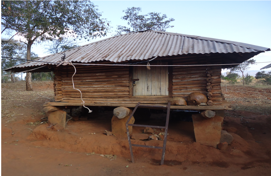
Appendix 4.7: storage structure- granary in Machakos county in kenya
